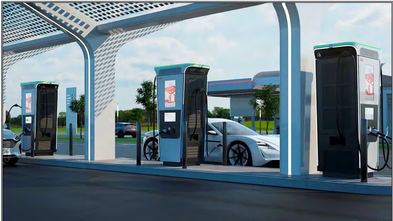
Example of DC Fast Charging with conventional pull-through service island
