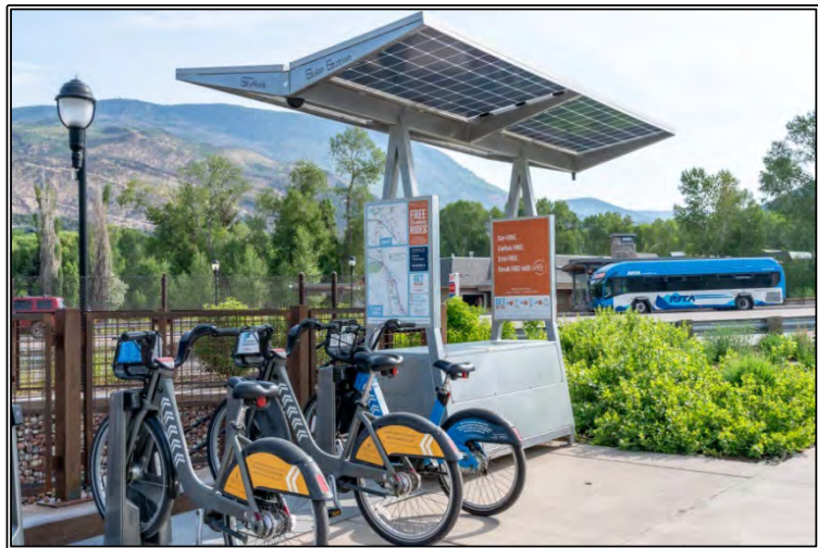
Shared E-Bike solar-powered, charging dock WeCycle / Sky Hook charging station, Basalt, Colorado
