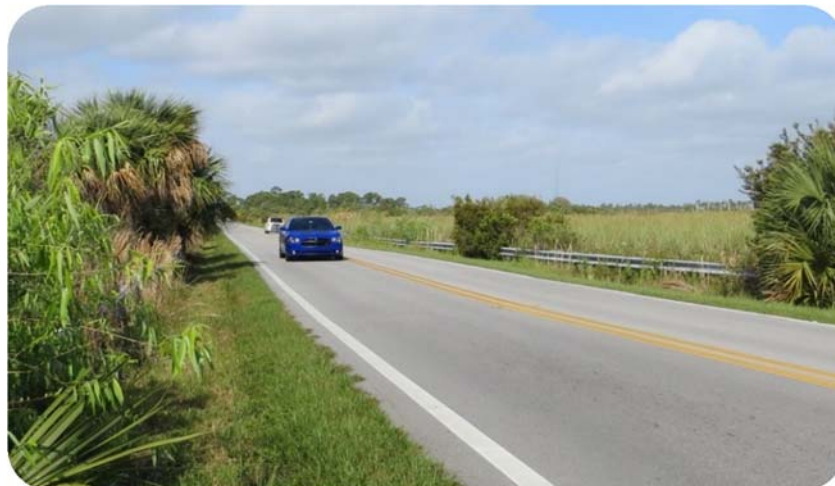
Figure 3.1 Two Lane Section from Segment C
