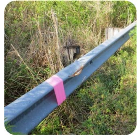
Figure 2.2 Damaged Guardrail
