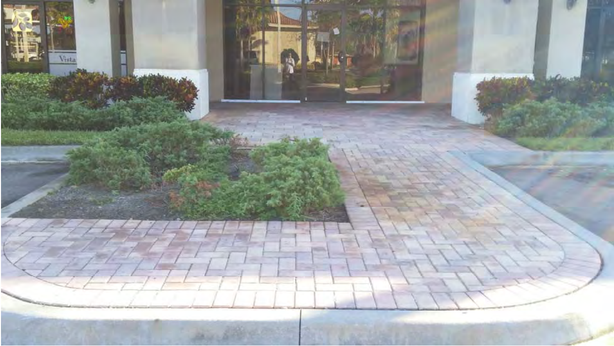
Figure 6: CocoVista Center Potential space for U Racks
