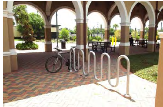
Figure 18: Fort Pierce Avenue D Bus Terminal
