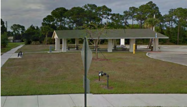
Figure 17: Port St. Lucie (Deacon Avenue) Terminal
