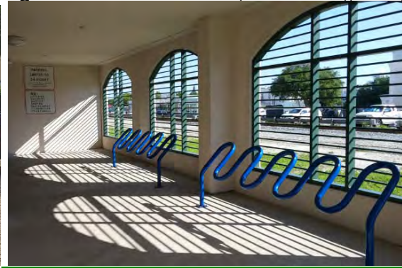
Figure 20: Fort Pierce City Hall Parking Garage
