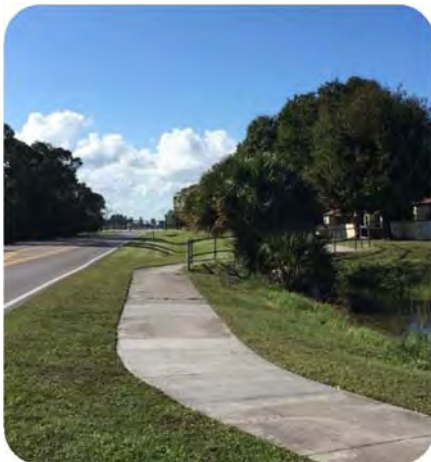
Figure 1.5 Sidewalk on North
