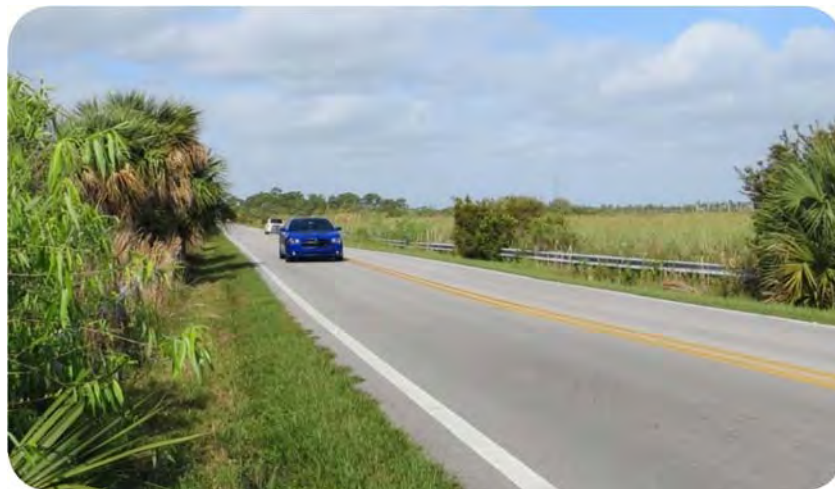
Figure 3.1 Two Lane Section from Segment C
