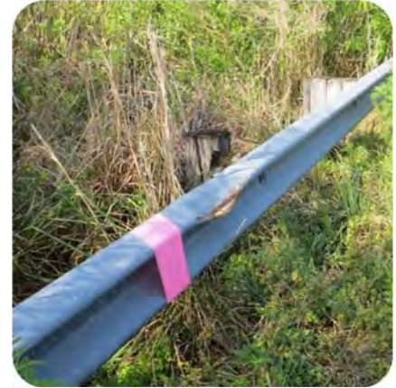
Figure 2.2 Damaged Guardrail
