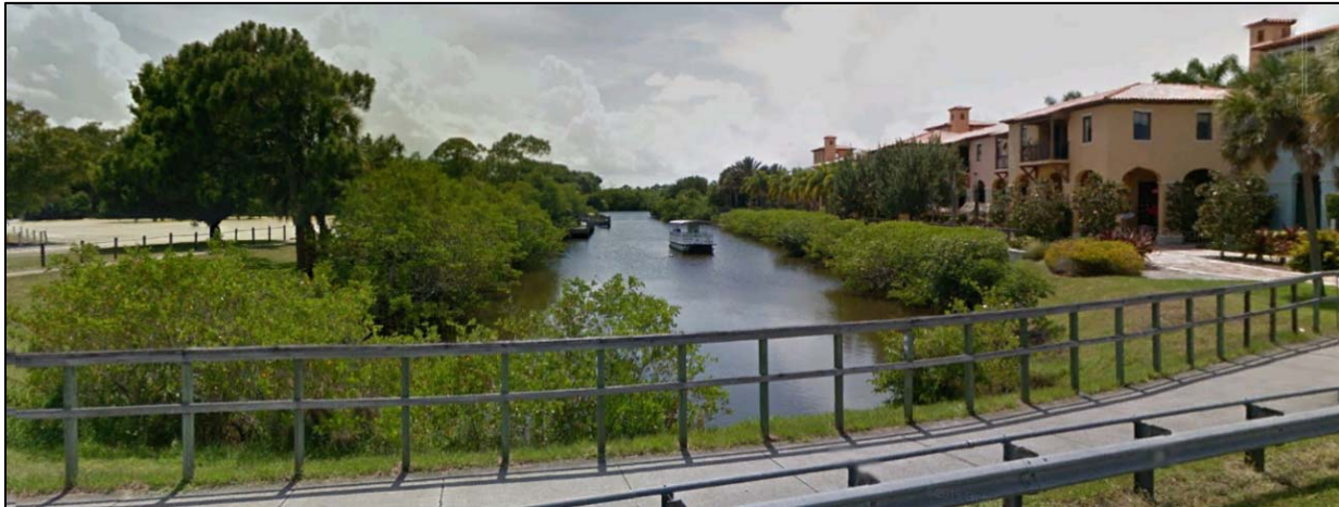
Figure 2: Veteran's Park at Rivergate - Port St. Lucie Riverwalk Boardwalk
