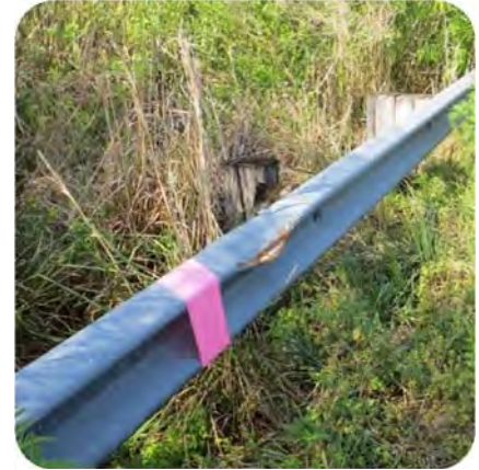
Figure 2.2 Damaged Guardrail
