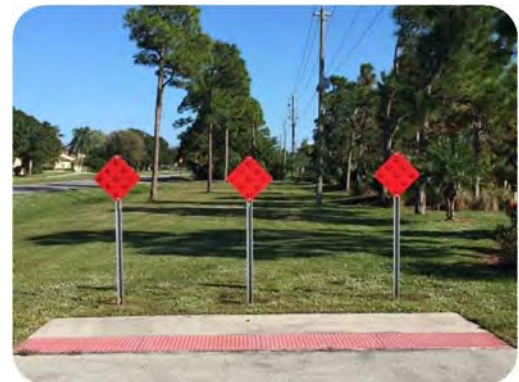
Figure 1.3 End of Shared Use Path
