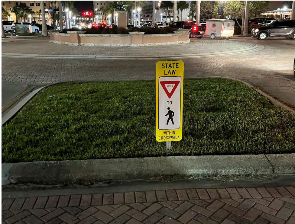
Exhibit 34: Yield to Pedestrians Sign at Roundabout Crosswalk
