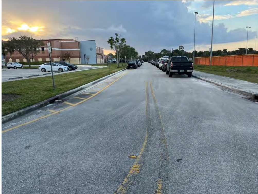
Exhibit 54: Vehicles Parked in No Parking Zone
