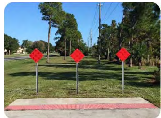
Figure 1.3 End of Shared Use Path
