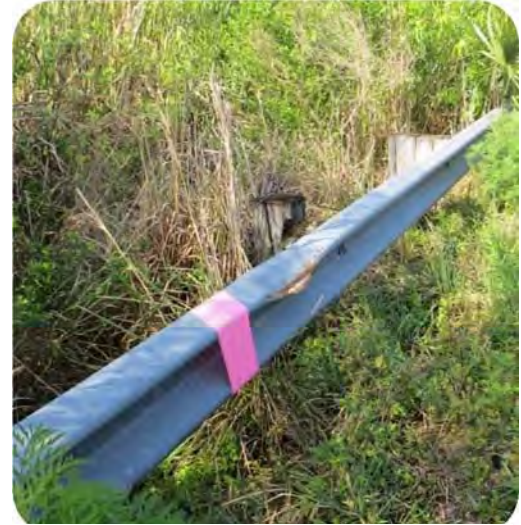
Figure 2.3 Damaged Guardrail
