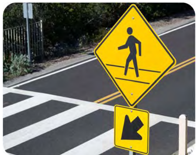
Figure 3.3 Example of Pedestrian Crossing on Green River Parkway
