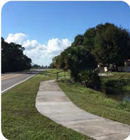
Figure 1.5 Sidewalk on North
