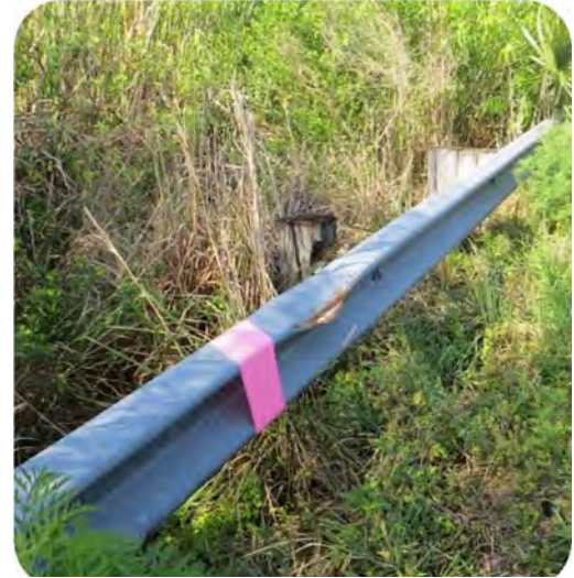
Figure 2.3 Damaged Guardrail
