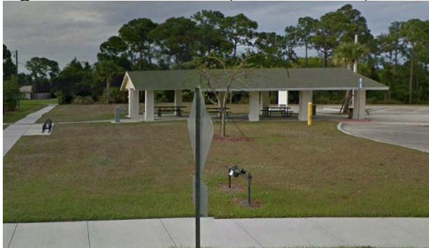
Figure 17: Port St. Lucie (Deacon Avenue) Terminal
