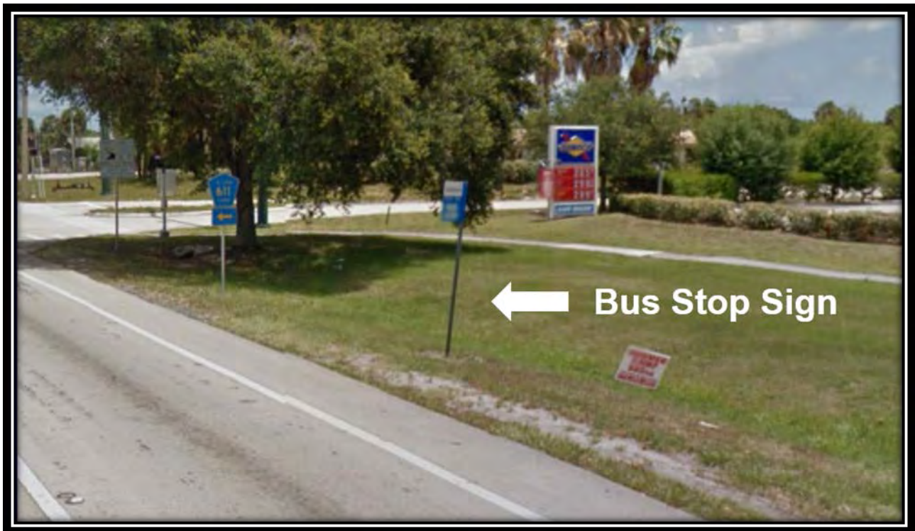
Figure 2 – U.S. 1/Edwards Road Northbound Bus Stop
