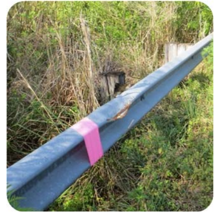
Figure 2.2 Damaged Guardrail
