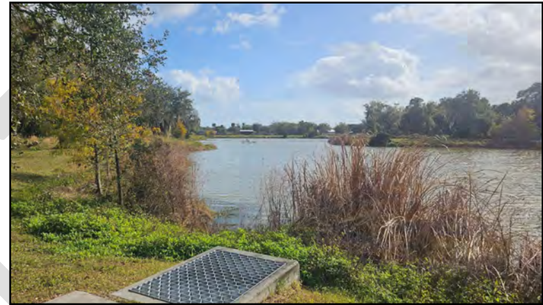
Citrus Hammock Preserve Water Retention Area
