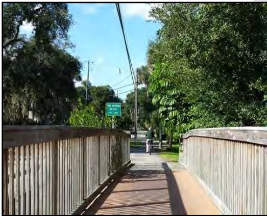
Clay-Duval Trail bridge
