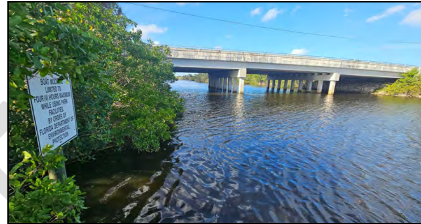
Prima Vista Bridge over St. Lucie River
