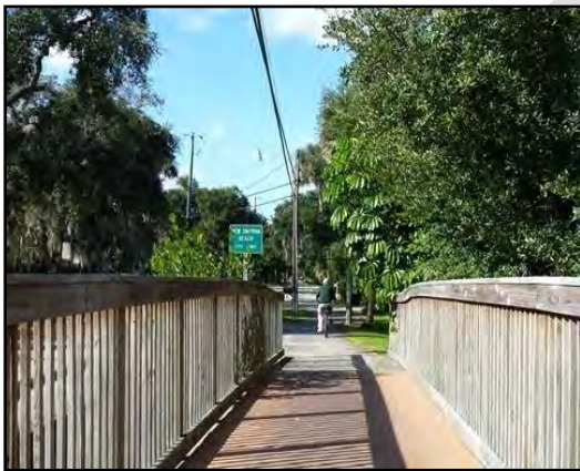
Clay-Duval Trail bridge
