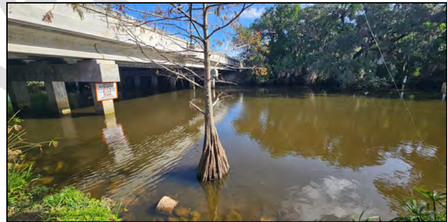
Midway Bridge at White City Park
