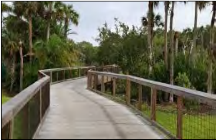
Gordon River Greenway Boardwalk
